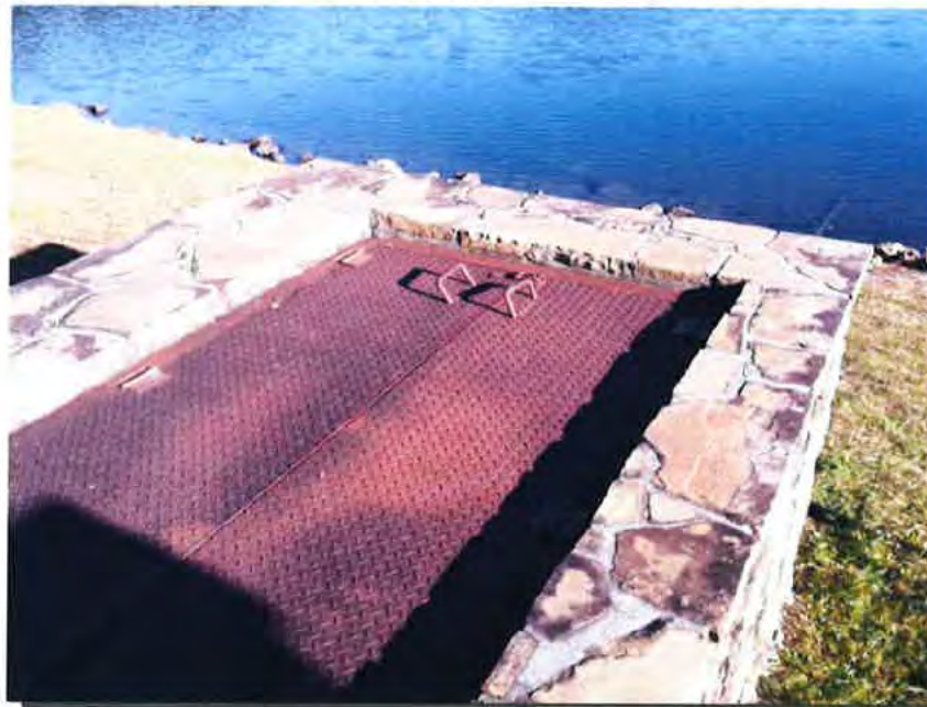
Photograph 2: View of the low-level valve box.
