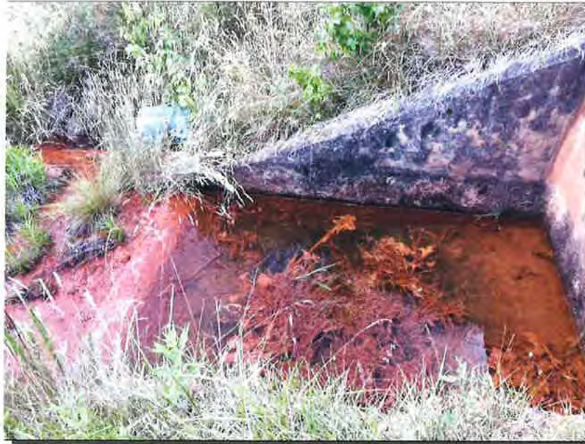
Photograph 3: Tail Water Creek, 2016 – Low-level drain outlet.
