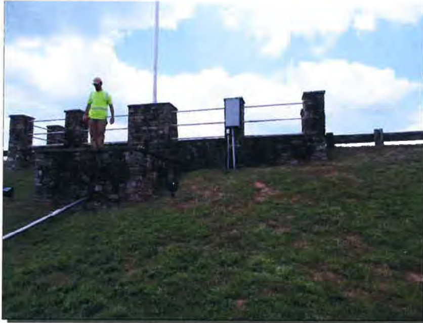
Photograph 1: View of the low-level valve box
